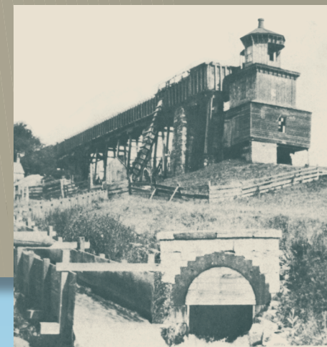
The Plane 9 West power house is seen above, while below water flows from the bypass trough on the left and the tailrace tunnel on the right.
